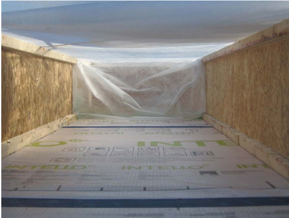
36" x 16" Roof Cavity
