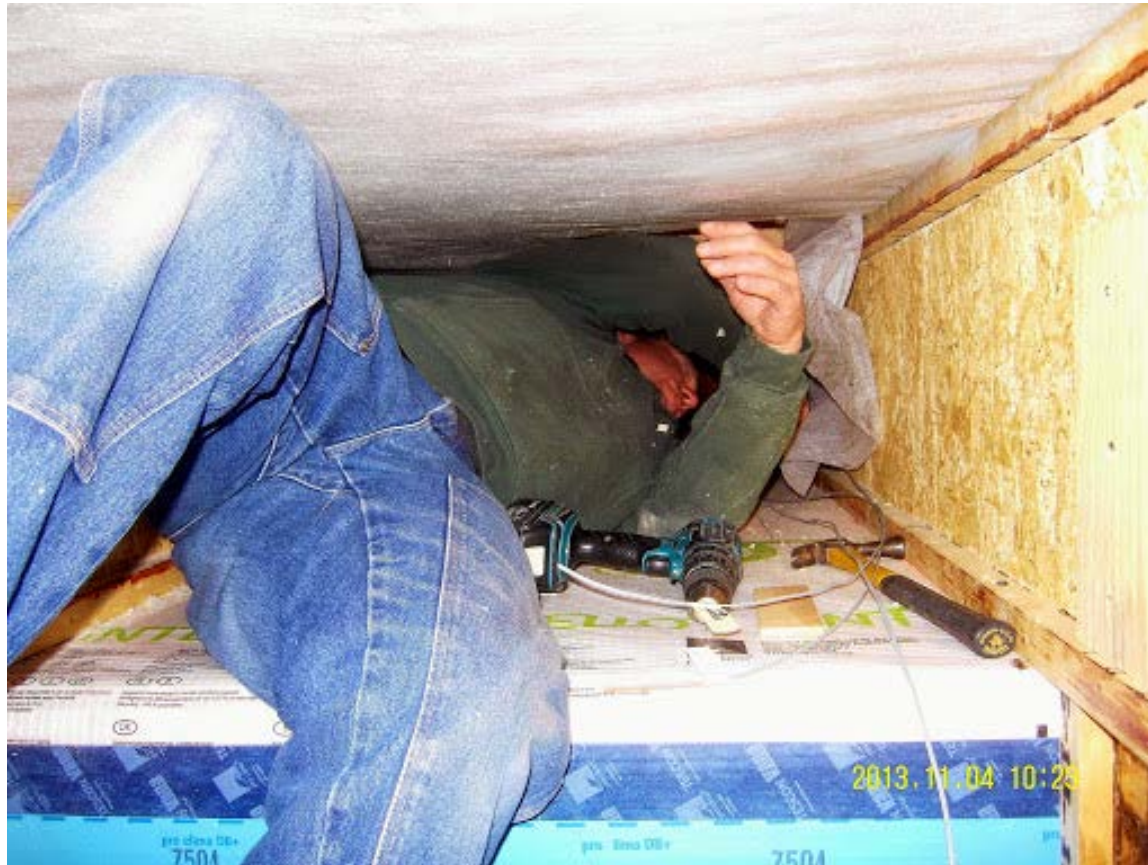
NE Roof Sensor, 60" up rake from North wall
