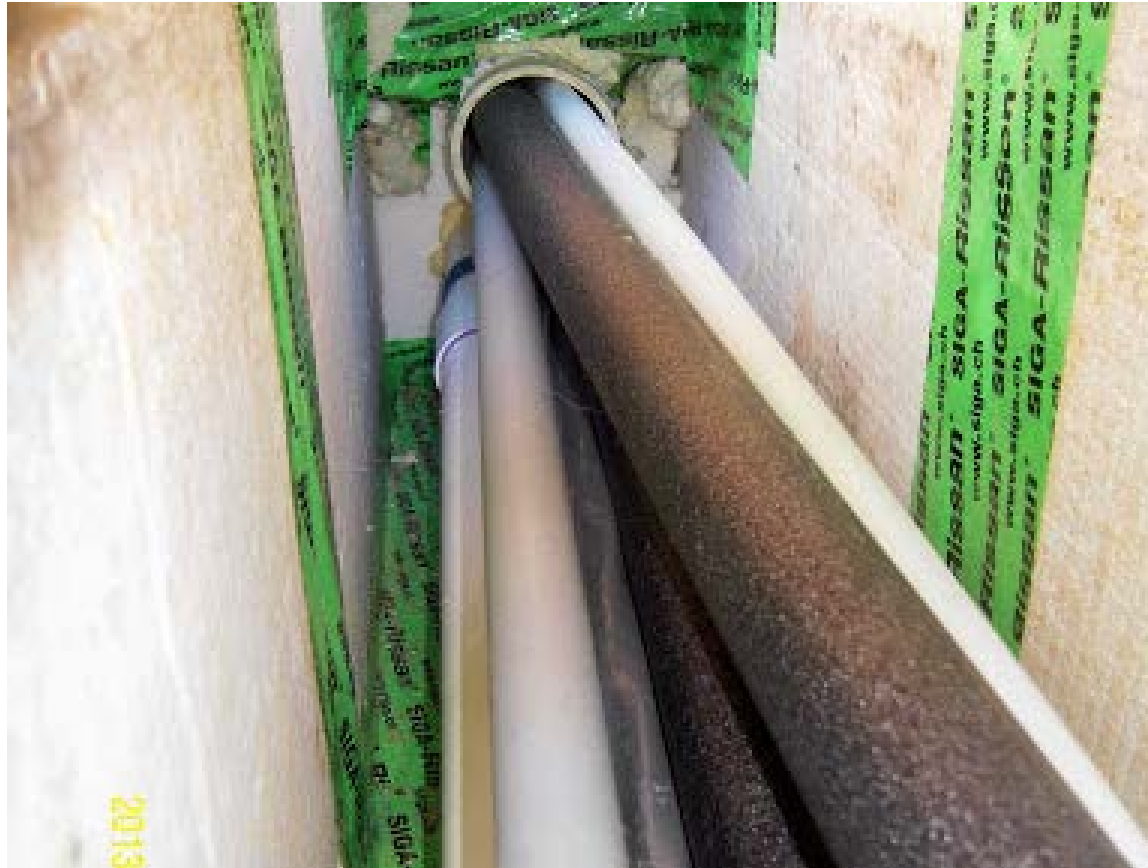
Utility Chase - Super Insulated-Air tight
