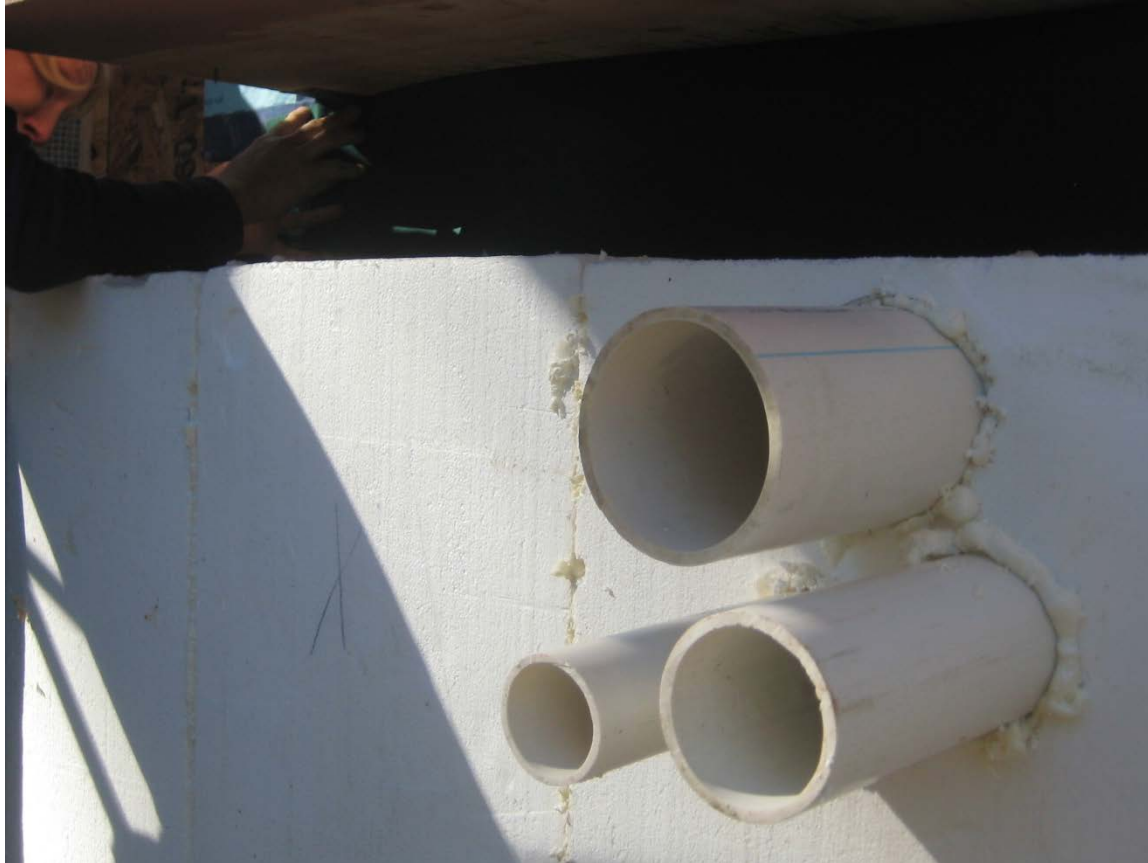
Completed Utility Chase Penetrations
